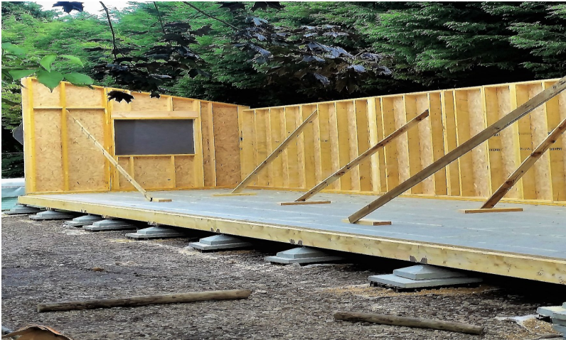
Kit going up. Note Plinths not included unless stated
